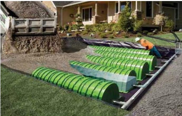
Figure 5–22 Project Precedent - Underground Infiltration Modules with Gravel Overlay
