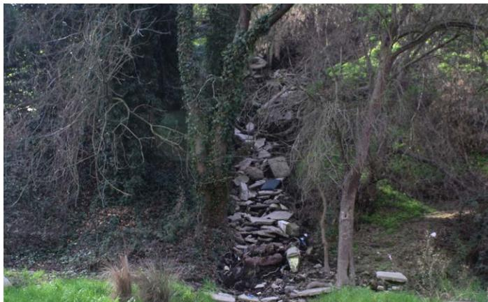
The outfall pipe is located just over the hillside at the 7th Street and Atchison Street (SR108) intersection. There is significant scour at the end of the outfall pipe (which is in poor condition) and an eroded channel has formed down to the river, with extensive sediment deposits where the flow path flattens out. The channel appears to have been filled with rock and rubble to provide erosion protection.
