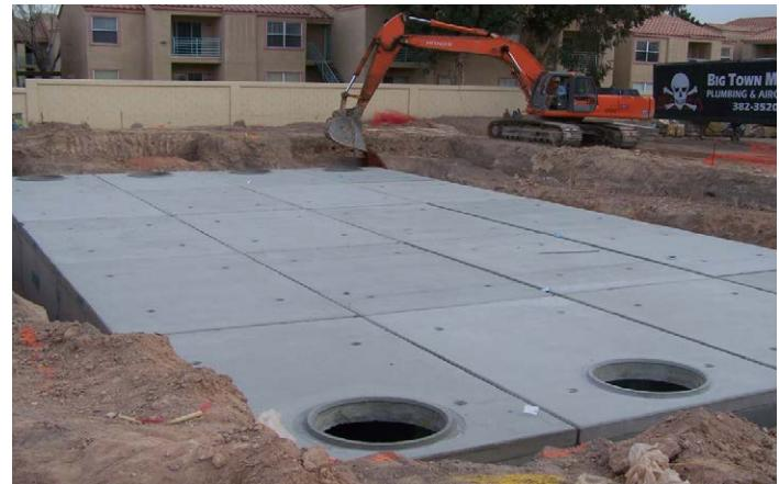
Figure 5–23 Project Precedent - Underground Infiltration Gallery with Access Ports (Las Vegas, NV)
