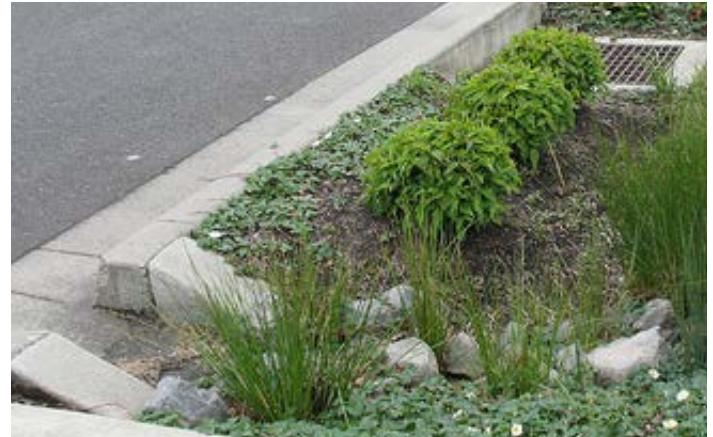
Figure 5–14 Project Precedent - Vegetated Swale with Concrete Inlet to Capture Drainage from Adjacent Roads
