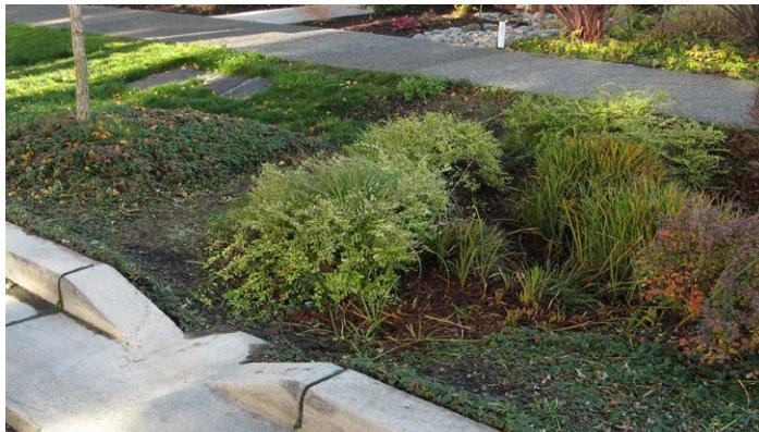
Figure 5–26 Project Precedent - Vegetated Swale with Concrete Inlet to Capture Drainage from Adjacent Road (High Point Seattle, WA)
