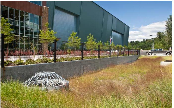
Figure 5–35 Project Precedent - Bioretention Basin with Overflow Structure (Seattle Seahawks Stadium, WA)
