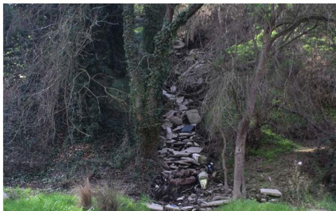
The outfall pipe is located just over the hillside at the 7th Street and Atchison Street (SR108) intersection. There is significant scour at the end of the outfall pipe (which is in poor condition) and an eroded channel has formed down to the river, with extensive sediment deposits where the flow path flattens out. The channel appears to have been filled with rock and rubble to provide erosion protection.
