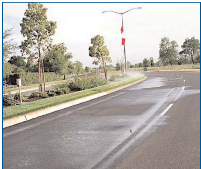
Watering the road is not water-wise.
