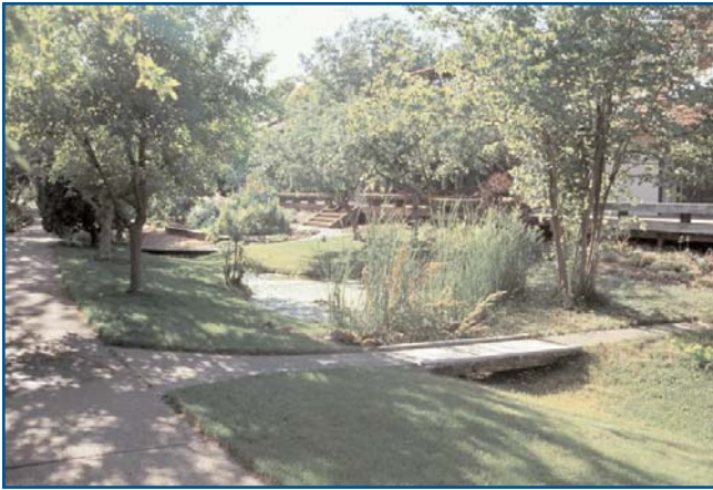
A network of open swales at the Village Homes development in Davis, CA, provides an aesthetic landscape as well as manages all stormwater on site.
