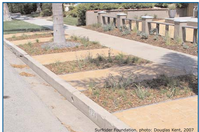
Pavers provide a permeable area for people to use when exiting or entering their car when it is parked along the street.
