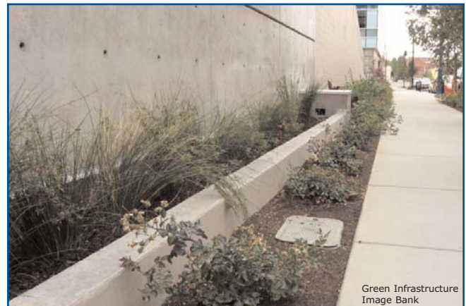
These planters in Emeryville, CA, are designed with overflow boxes and underdrains.
