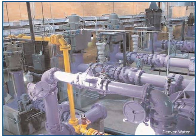
Purple pipe system
