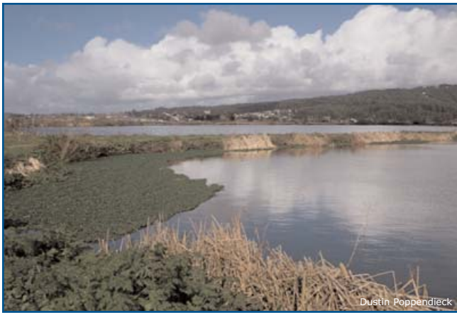
Arcata Wastewater Treatment Plant oxidation ponds
