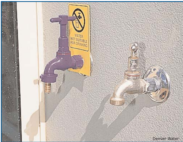
Recycled water is carried in purple pipes to ensure it remains separate from potable water sources.
