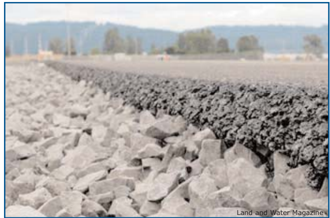
The Port of Portland Terminal 6 project used a combination of porous pavement laid over a coarse aggregate base and vegetated swales to handle 100% of the stormwater generated on a 51-acre redevelopment site.
