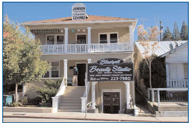
Mixed-use building in Downtown Jackson
