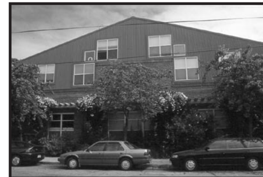
Avalon Garden Senior Apartments (top), in Emeryville, California, was developed by Avalon Senior, L.P. and the East Bay Asian Local Development Corp. as very low and low income housing for seniors. In the same city, an old industrial building (bottom) was converted to the Doyle St. CoHousing project.
