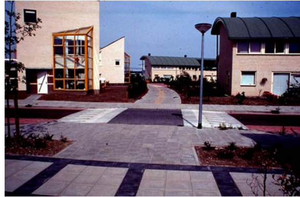
In Grand Junction, Colorado this flat-topped speed table (above) creates a level surface for pedestrian and trail crossings. Speed tables, such as this one, can be applied as the only traffic calming feature. As shown below speed tables can also be used in combination with medians, curb extensions and other treatments.
