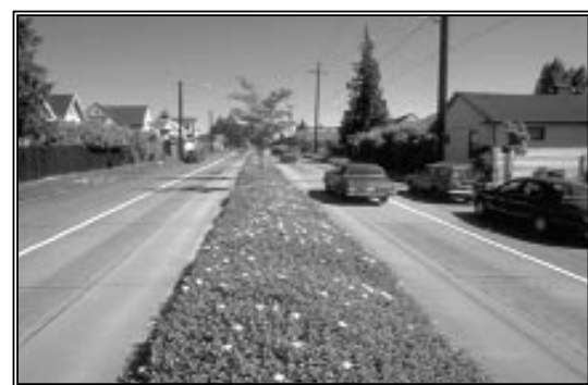
Used in combination with bike lanes, this landscaped median in Seattle, Washington, converted this fast street to one lane in each direction that is pleasant for walking, bicycling and driving. The prudent driver sets the speed for all.
