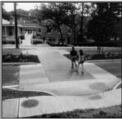
A refuge island with speed table can be an excellent traffic calming and safety element near schools.
