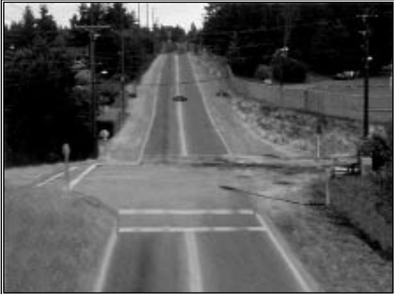
Grandview Avenue in University Place, Washington. Grandview was experiencing speeds in the low 40s before traffic calming treatments were implemented. With the addition of curbs, sidewalks, bike lanes, trees, medians, and a roundabout, speeds were reduced to the low 30s.
