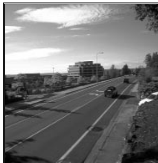
This section of Lake Washington Boulevard in Kirkland, Washington, was narrowed from four lanes to three. The conversion has created a smoother flow rate, addressed capacity issues, improved safety, and made way for a bike lane – which also provided a buffer for pedestrians.
