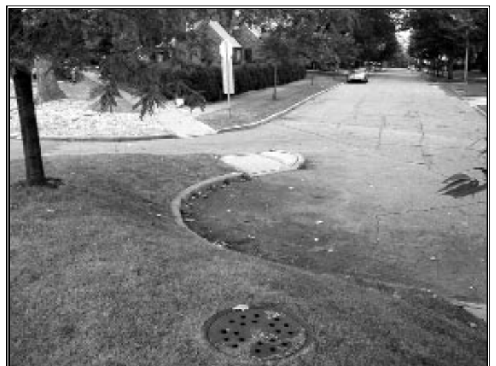
The partial street closure here permits a low speed exit only. Emergency fire and medical responders can still enter. Pedestrians and bicyclists have full access.
