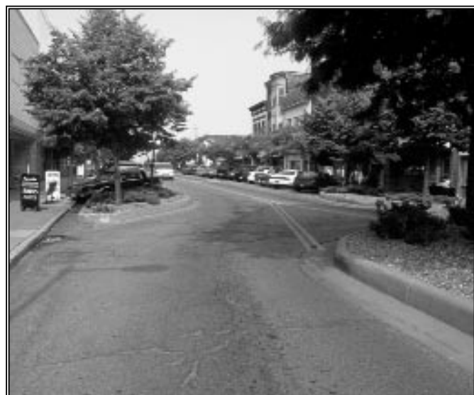
Chicanes can be used on streets with or without sidewalks. These chicanes narrow this Main Street to two lanes and require traffic to move slowly. This style of chicane can easily handle 5,000 to 10,000 vehicles per day.
