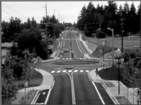
Grandview Avenue in University Place, Washington. Grandview was experiencing speeds in the low 40s before traffic calming treatments were implemented. With the addition of curbs, sidewalks, bike lanes, trees, medians, and a roundabout, speeds were reduced to the low 30s.
