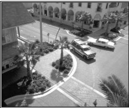
Bulbouts at an intersection in Venice, Florida, shorten the crossing distance for pedestrians and make drivers travel more slowly around corners.
