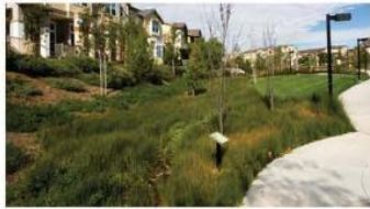
Bioretention areas are among the most common LID techniques implemented, often in highly visible locations, and can be a valuable educational opportunity especially if signage is installed illustrating function, intent, or native plants.
