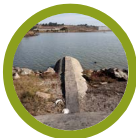
Outfall Retrofit/ Replacement
