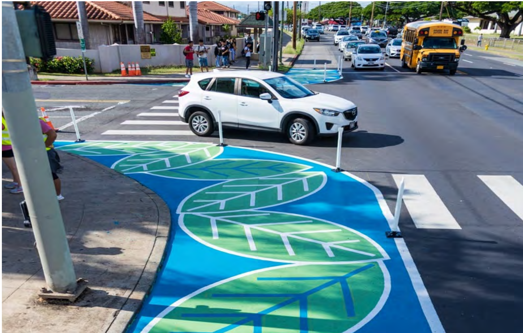
Example of quick-build curb extension
